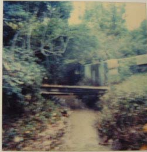
Looking D/S From culvert 11-22-82
